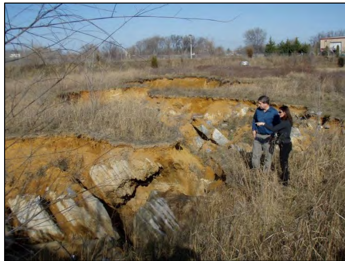
Sinkhole and retention pond collapse, Frederick MD. Photo by Dan Doctor.
