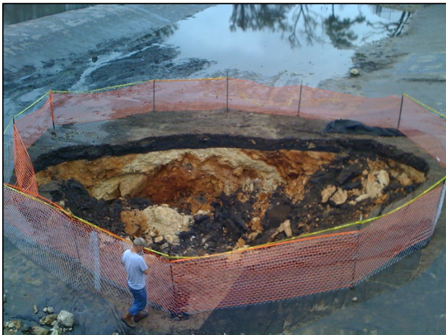
Cover-collapse sinkhole in the Edwards Formation within a stormwater retention pond, Austin Texas. Left photo taken soon after collapse, right photo showing rock fill and concrete plug. Photo by BSEACD.
