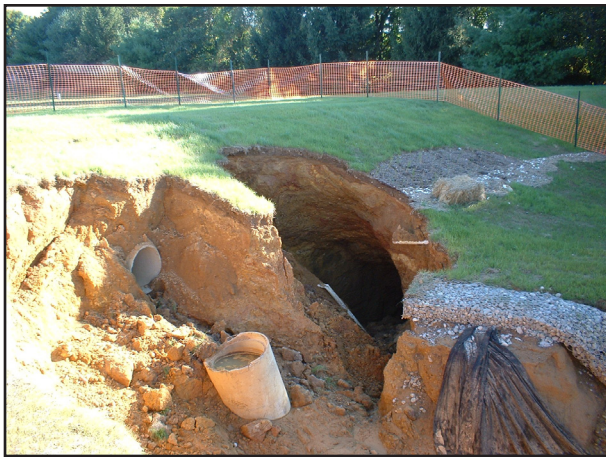
Sinkhole collapse along a stormwater line. Photo by Joe Fischer.
